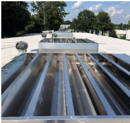
MatrixVent installed at peak, blades perpendicular to peak
