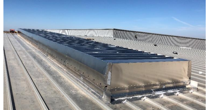
MatrixVent installed downslope, blades parallel to peak.
