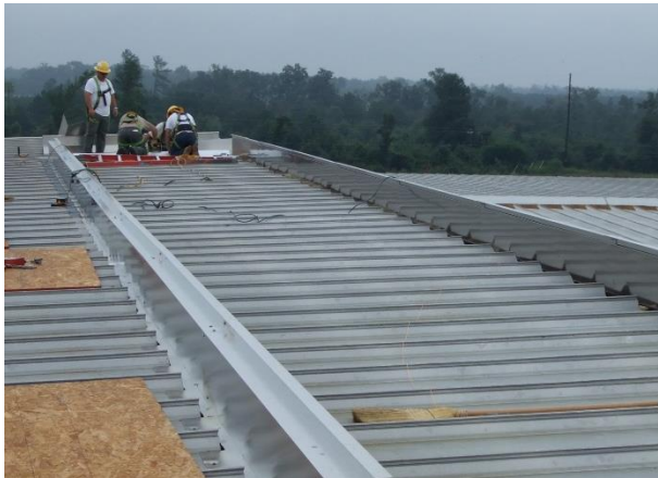
MatrixVent assembled directly on the roof of the facility
