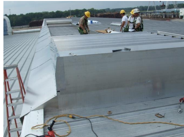
MatrixVent assembled directly on the roof of the facility
