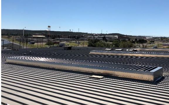
MatrixVent installed downslope, blades parallel to peak.
