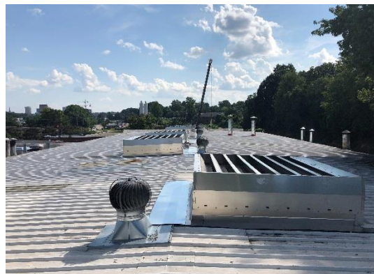
MatrixVent installed onto curb on membrane roof
