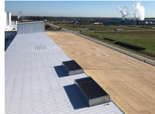
MatrixVent installed at peak, blades perpendicular to peak
