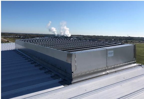
MatrixVent installed at peak, blades perpendicular to peak
